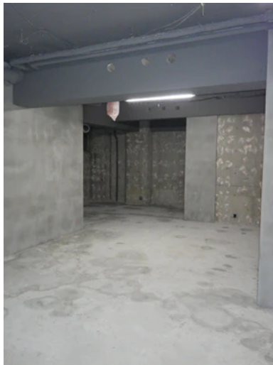
Restored to original condition
